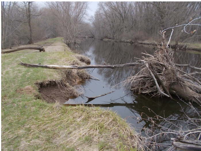
Photo of dike damage on Rice Lake River
